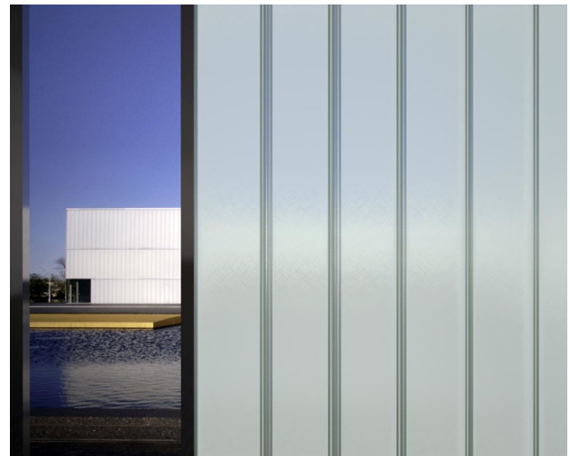
Channel glass wall with Thermolight 100 insulation
