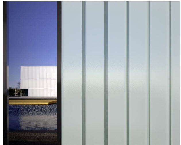
Channel glass wall with Thermolight 100 insulation
