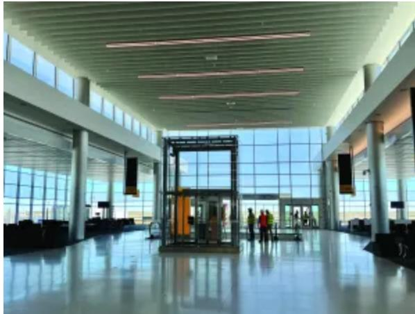
***Seeking to limit visual obstruction, project architects sought to create a clear glass elevator shaft with the bare minimum of visible hardware.***
