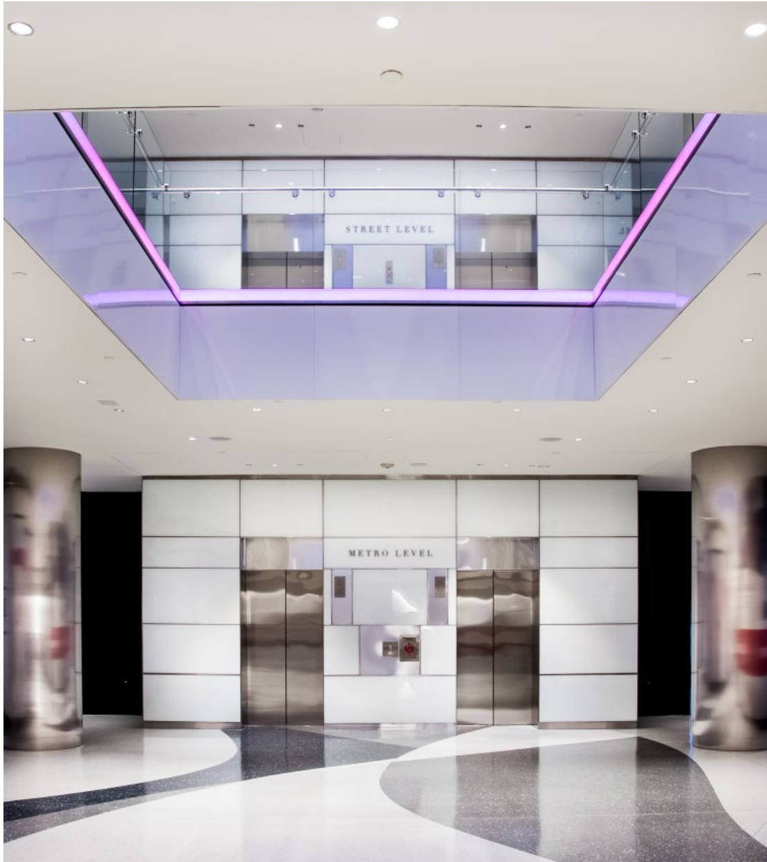
Chevy Chase Pavilion, Washington, DC. White back-painted glass [Picture courtesy of Bendheim LLC].
