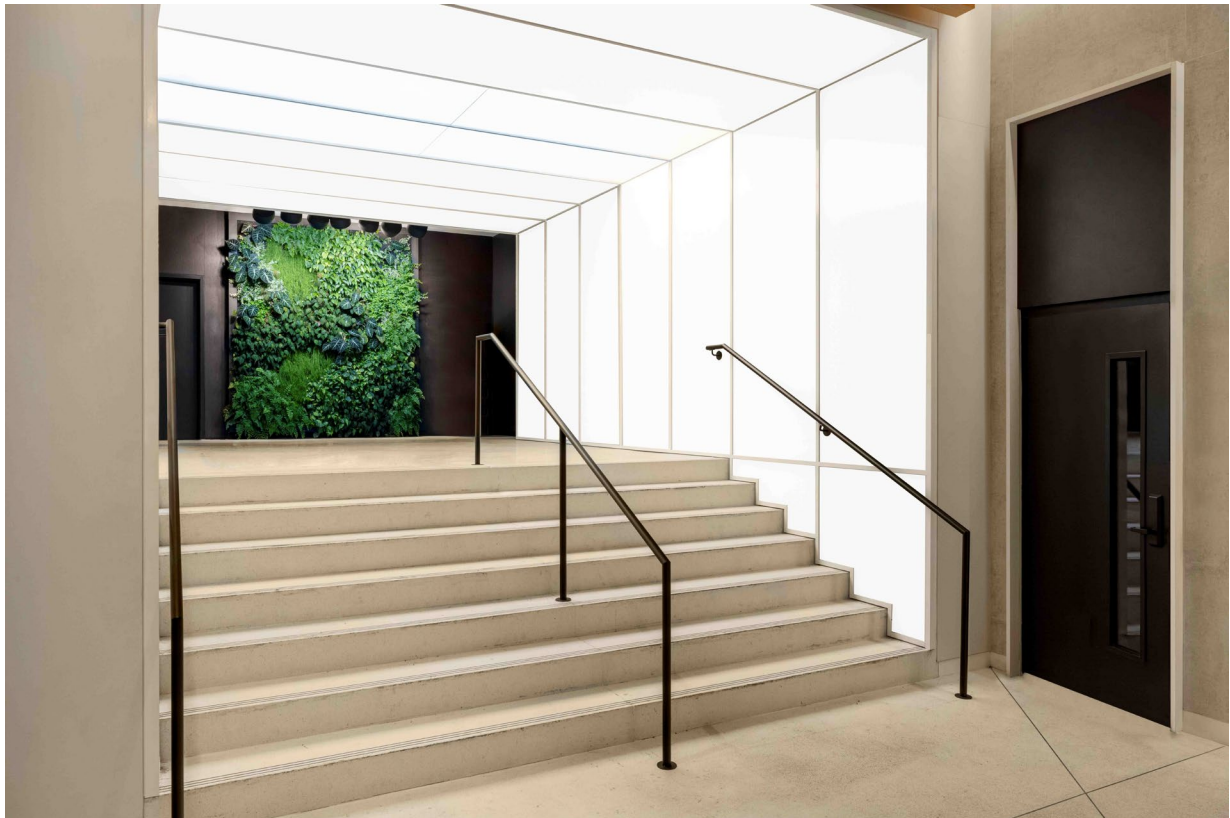
200 Varick St., New York, NY. Laminated glass with white EVA [Picture courtesy of Bendheim LLC].
