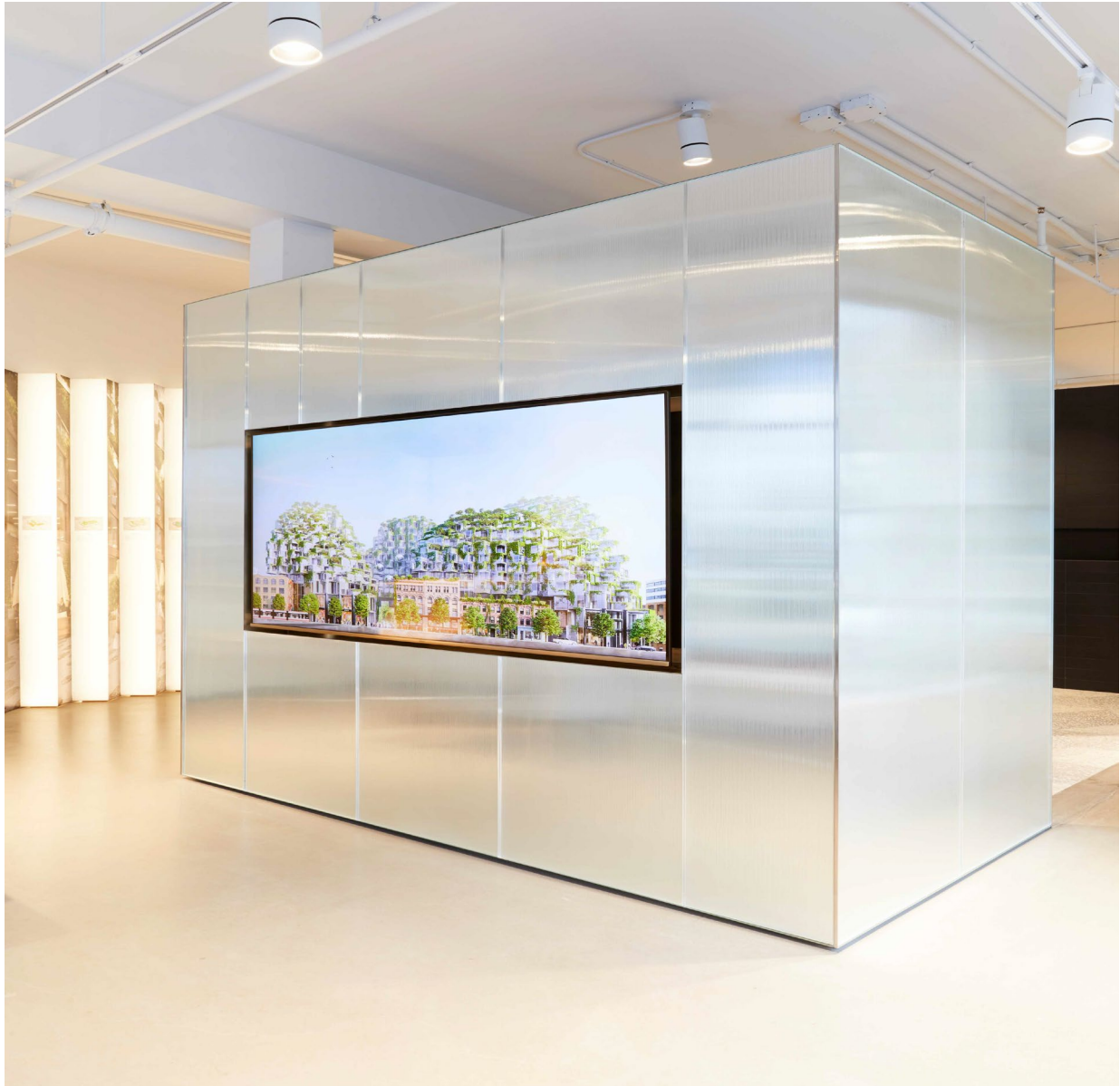
King Street Condo Tower, Toronto, ON. Textured glass laminated to mirror [Picture courtesy of Bendheim LLC].
