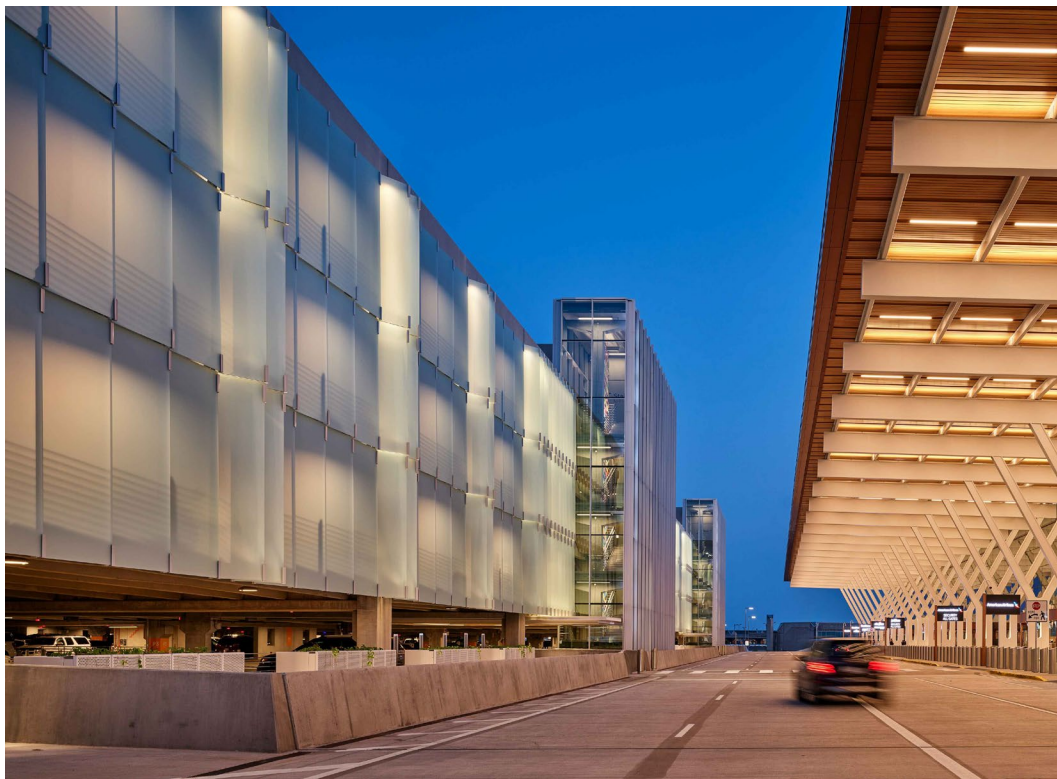
Kansas City International Airport parking structure, Kansas City, MO. Laminated etched glass [Picture courtesy of Bendheim LLC].
