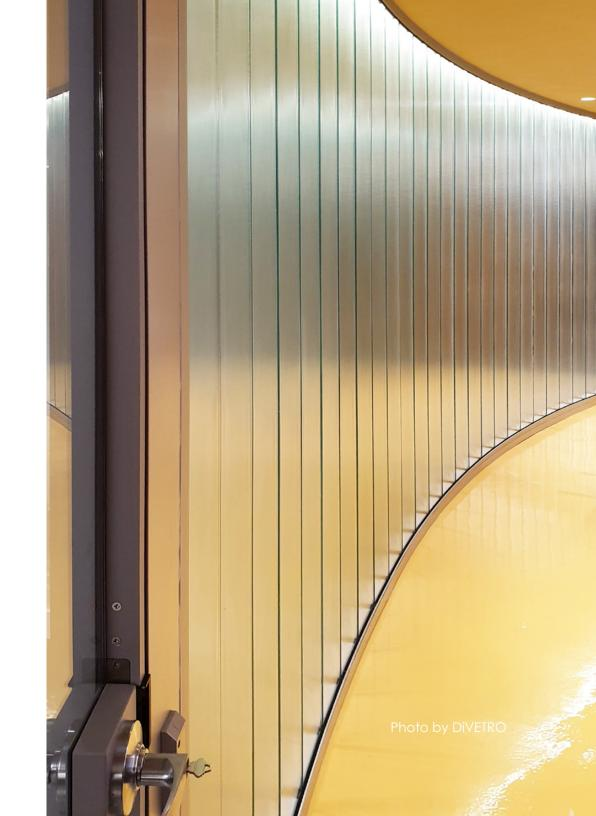
channel glass partition wall. The daylight-friendly, privacy-friendly glass wall simultaneously divides the space and maintains a sense of openness and connectivity.
