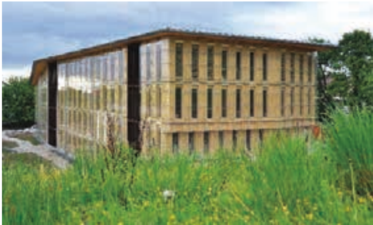
Drained and back-ventilated glass rainscreen features horizontally and vertically overlapping safety laminated glass panels at this 1300-m 2 (14,000-sf) commercial building in Freiburg, Germany.
