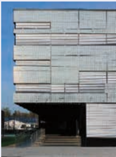
Drained, back-ventilated rainscreen system features white fritted glass at Sebastian Lotzer Secondary School in Memmingen, Germany.
