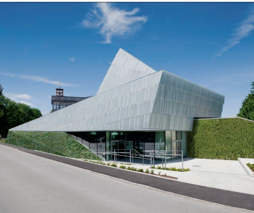
Rif Community Centre (Salzburg, Austria) features a, sloped, ventilated glass rainscreen with vertically and horizontally overlapping etched glass panels.
