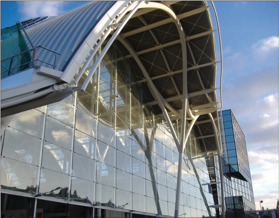
The train station in Orleans, France, features a glass rainscreen with horizontally overlapping, tempered panels.
