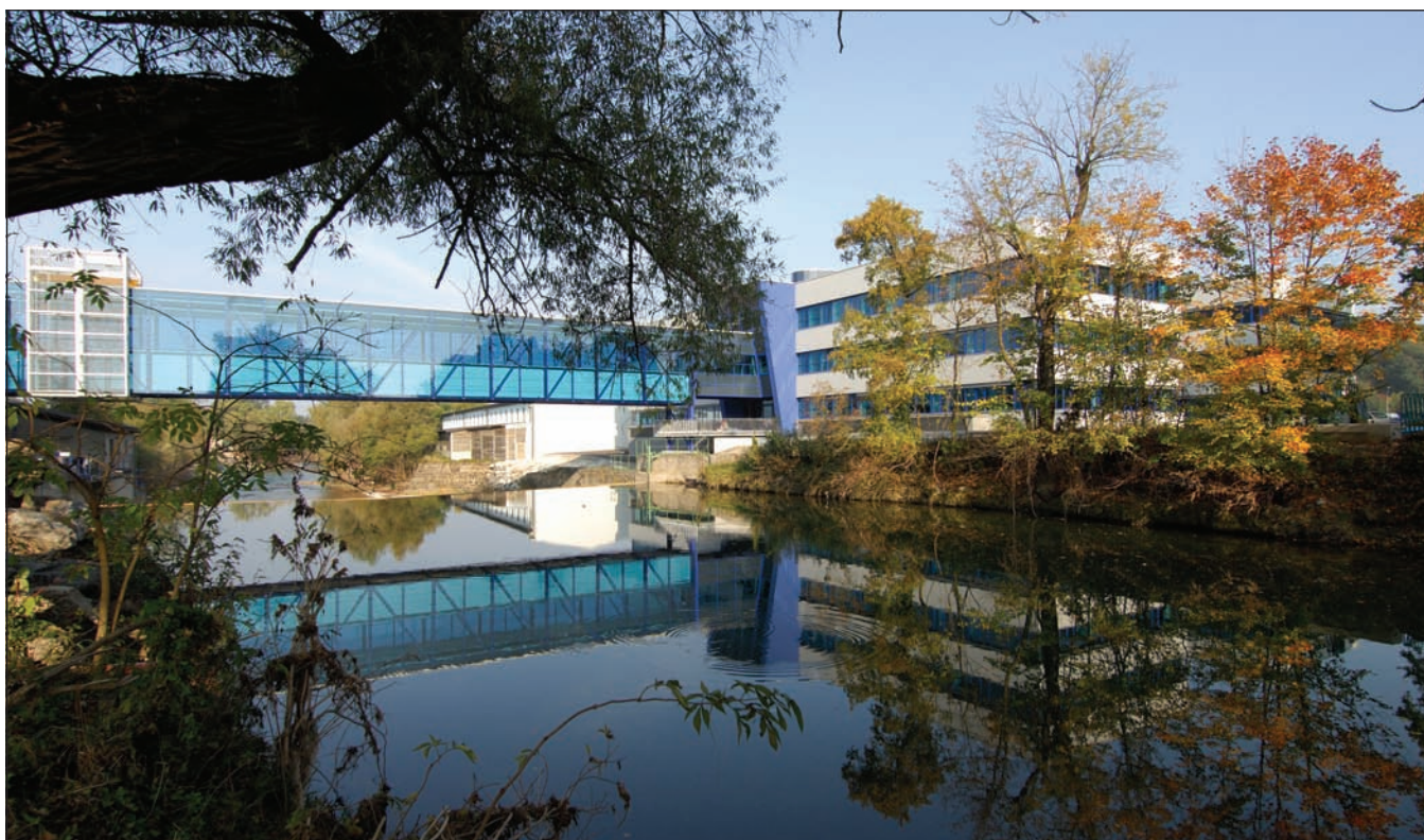
At the Zizala Lighting Systems in Wieselburg, Austria, the ventilated glass rainscreen system features compression glass fittings and coloured glass to create an enclosed walkway between two commercial buildings.
